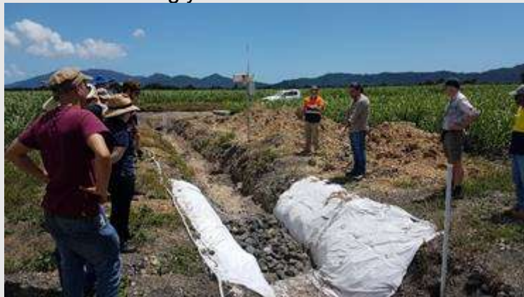
A denitrifying bioreactor site built into the base of a drainage channel in Queensland
