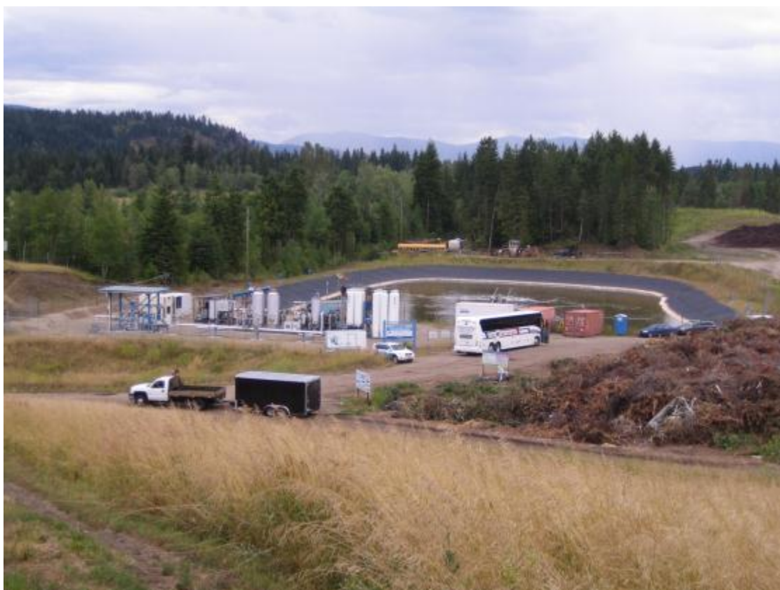
Figure 1. Landfill leachate pond and a prototype plant to capture and pressurise methane gas for commercial use, at Salmon Arm in BC, Canada.
