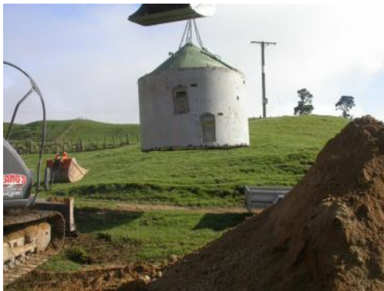
Fig. 1: Top section of the Spydia lifted out of the ground.
