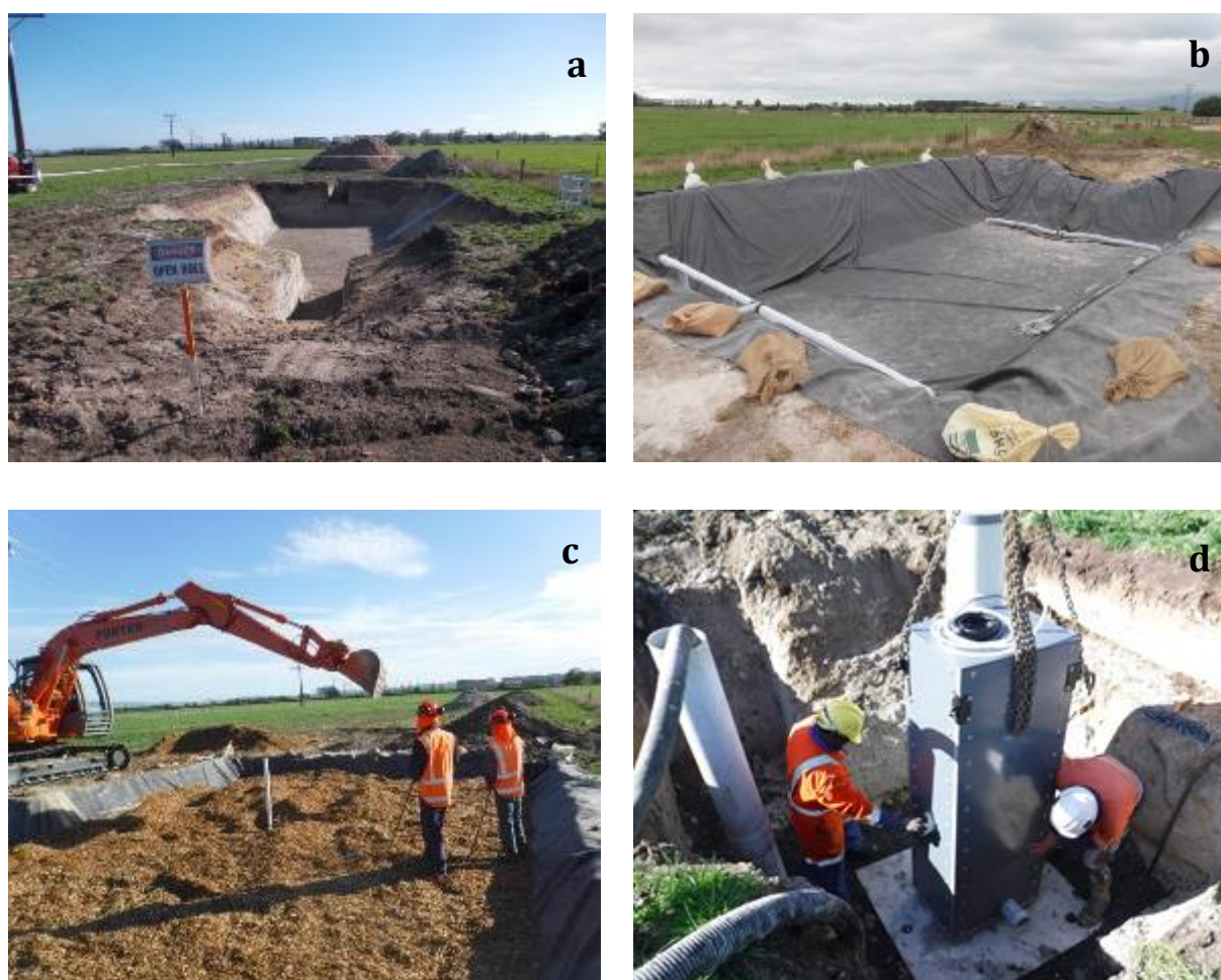
Figure 1 Construction of the denitrifying bioreactor: a) excavation of the pit, b) geomembrane lining, c) filling with woodchips, d) control box installation.
